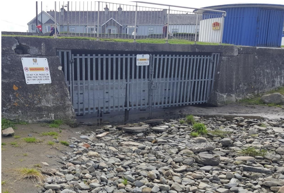
Figure 2-20: Victoria Outfall with weir board in place
