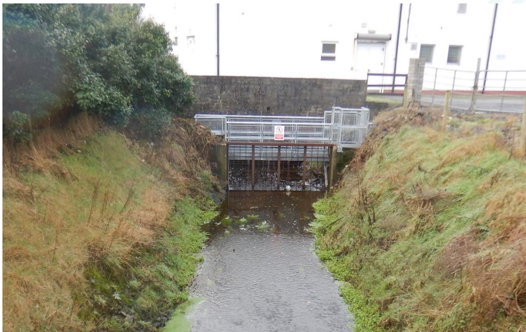
Figure 2-21: Trash Screen on Atlantic Stream
